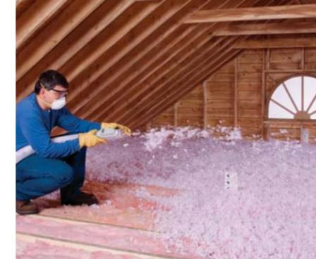
**The AttiCat® Expanding Blown-in Insulation Machine conditions the AttiCat® Expanding Blown-in PINK FIBERGLAS™ Insulation by breaking it up and fluffing it.**
